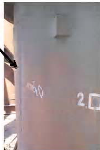
Figure 2. Geometrical deviations: – metal chimneys: a) convexity/dimple on the shell; b) eccentricity; – gas exhaust trunks: c) concavity of a shell; d) withdrawal of edges.
