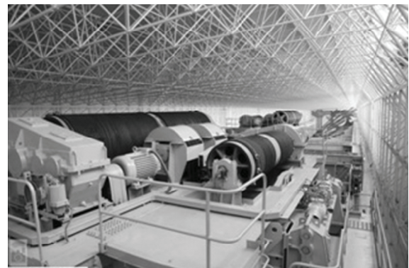
Figure 2. Turbine room span – Bureyskaya Hydropower Station (size covered 150.0×28.5 m).
