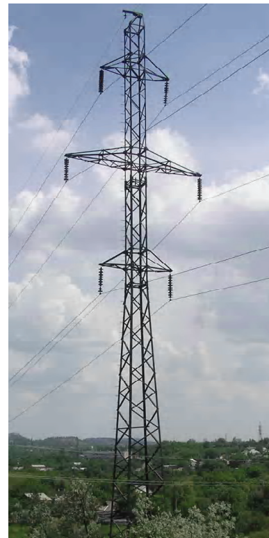
Figure 2. The general view of the intermediate support P110-6.
