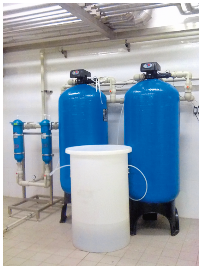
Figure 8. Water treatment station for a boiler room
