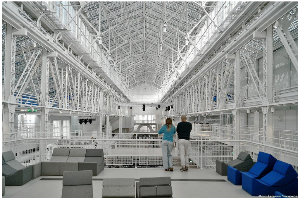
Figure 5: Main hall of HPP-2
