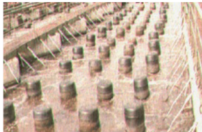
Figure 5. Layout of floats – bioreactors in the section of the Korsun river
